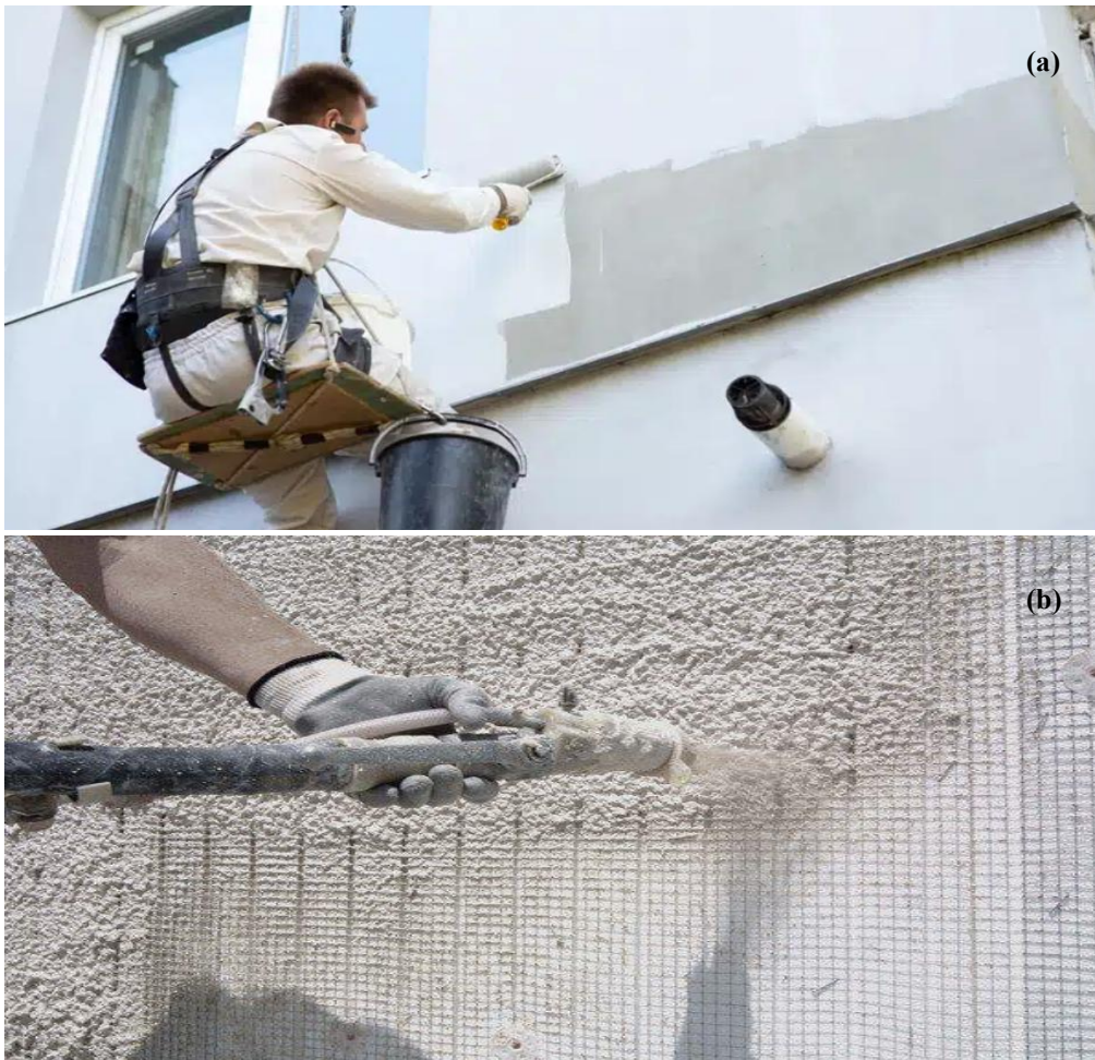
Figure III.22. Types of insulating coatings. (a): Thermal insulating paint, (b): Polystyrene-based render. Source : (Rhea Habitat, 2024; Isolation-Thermique, 2025)
