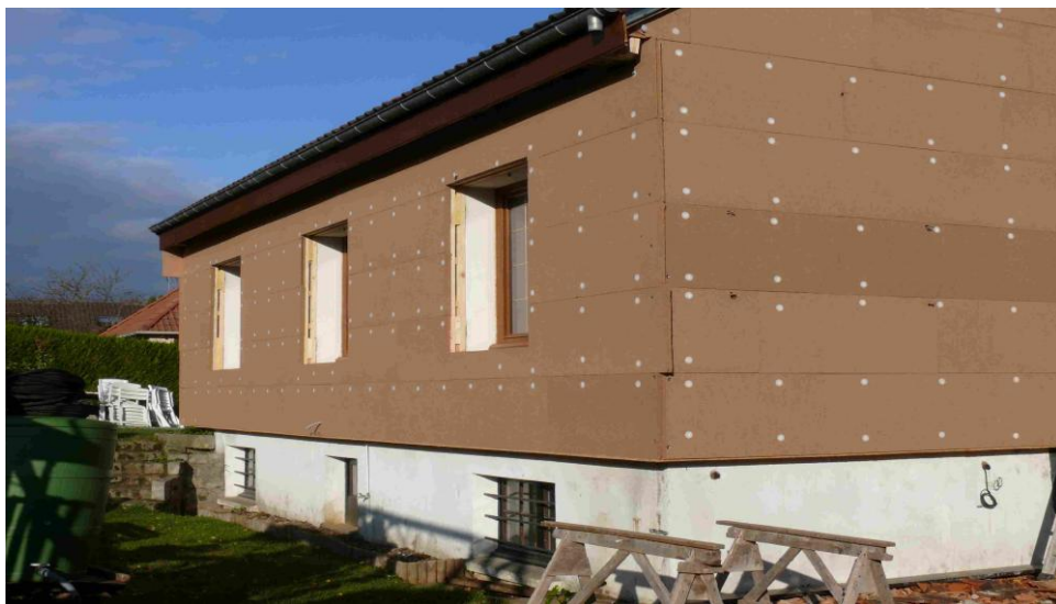
Figure III.17. ETI with wedge-laminated wood fiber panels. Source : (Dieumegard , 2016)
