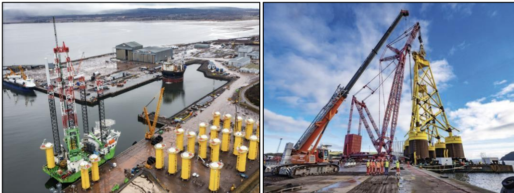
Figure 8 – Loading, deployment and installation of equipment
