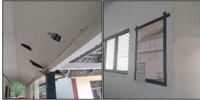
Fig. 4. Building condition of SDN Tamanjaya 2: broken ceiling (top) and use of duct tapes to replace picture frames to minimize hazard during earthquakes.
