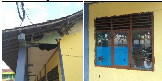
Fig. 2 Building condition of MTs Masyariqul Anwar: broken ceilings (top) and windows without trellises (bottom)
