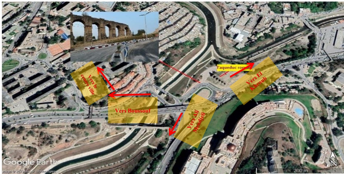
Fig 15. Djenane Zitoune interchange (Roman arches)
