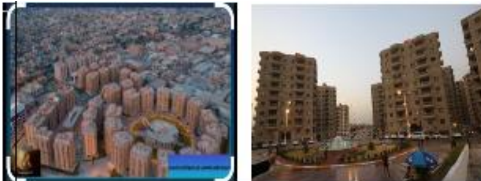
Figure 7. Several views of Al-Ayadi Residential Complex.
