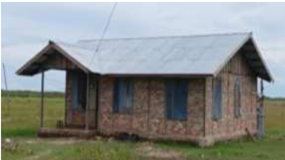
Fig. 2. Wooden House Structure
