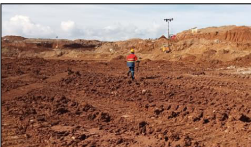
Fig. 8 Cut and Fill Topography Measurement
