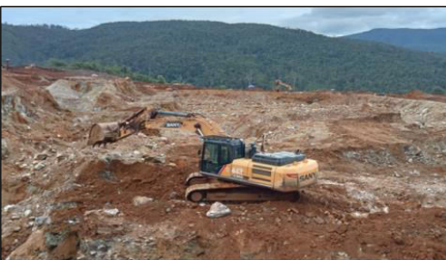
Fig. 7 Cut and Fill Process
