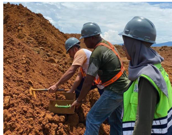
Fig. 2. The sampling process at the Bicoli stockpile
