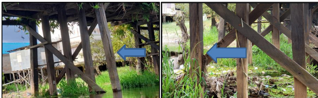
Figure 5. Tampa Bridge Condition during Investigation
