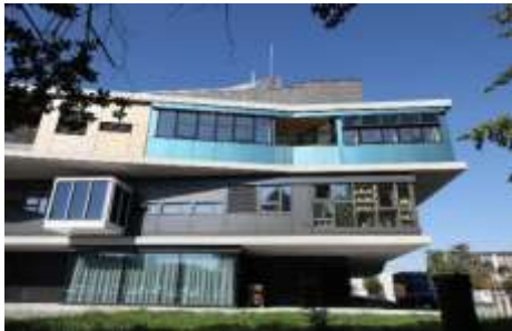
Fig. 4. STC in Nest Solace building, Switzerland [9]
