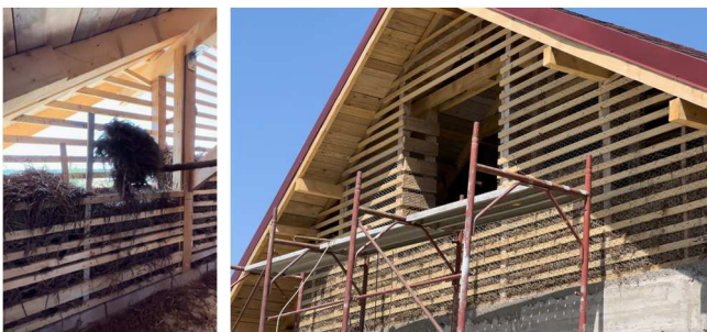
Fig. 4. The unheated attic walls filled with straws, previously treated for fire safety
