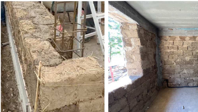
Fig. 3. External and internal walls made of adobe
