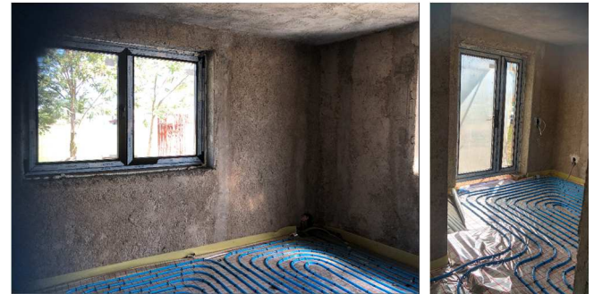
Fig. 5. Windows, doors and underfloor piping
